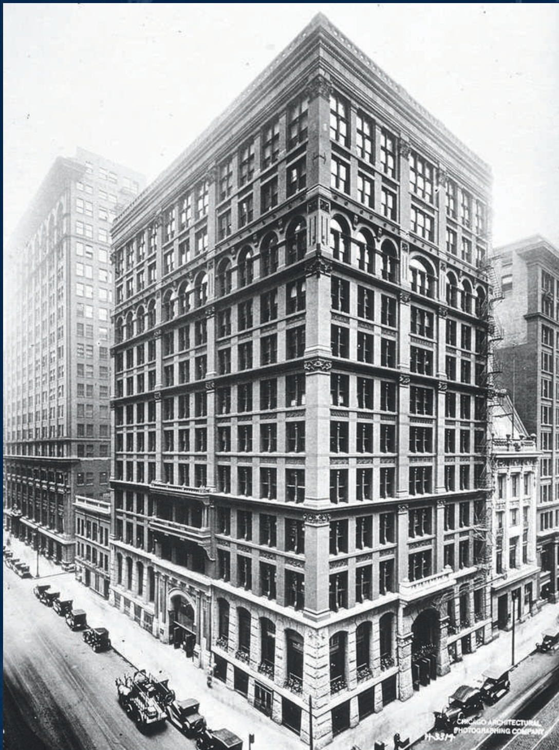
Home Insurance Building, Chicago (1870)
